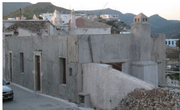
The house where Rosa was born. It was under renovation.
